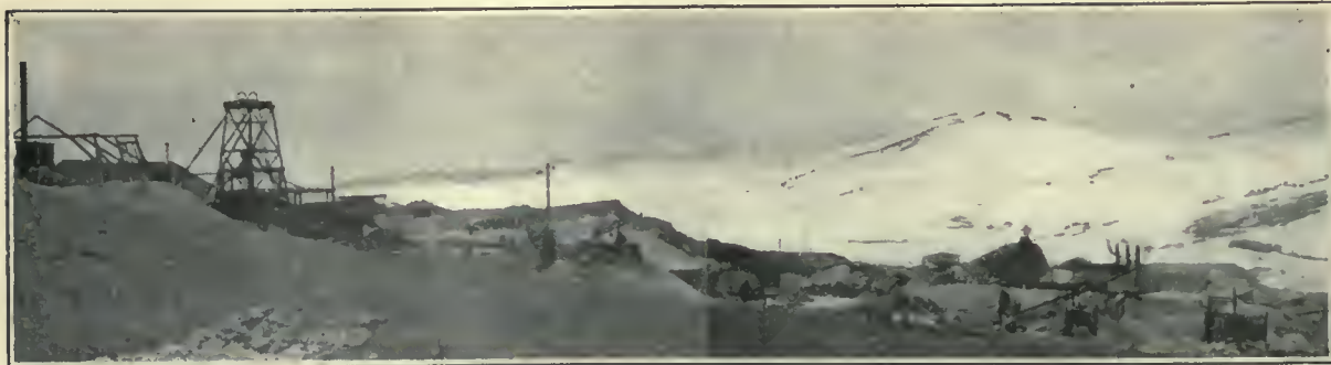
PANORAMA OF THE PODEROSA MINING COMPANY PROPERTY AT COLLAHUASI, CHILE. SHOWS THE SAN CARLOS AND PODEROSA HEAD-FRAMES AS WELL AS DUMPS, HAND-JIGS, AND OTHER HAND CONCENTRATING DEVICES.
